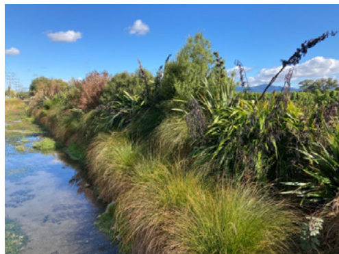
Two-stage channel with Carex secta planted on first level and flaxes and trees on the top level
