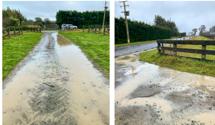
Water and sediment flowing down a driveway, exiting the vineyard and flowing down the road to a nearby drain which then enters a stream.
